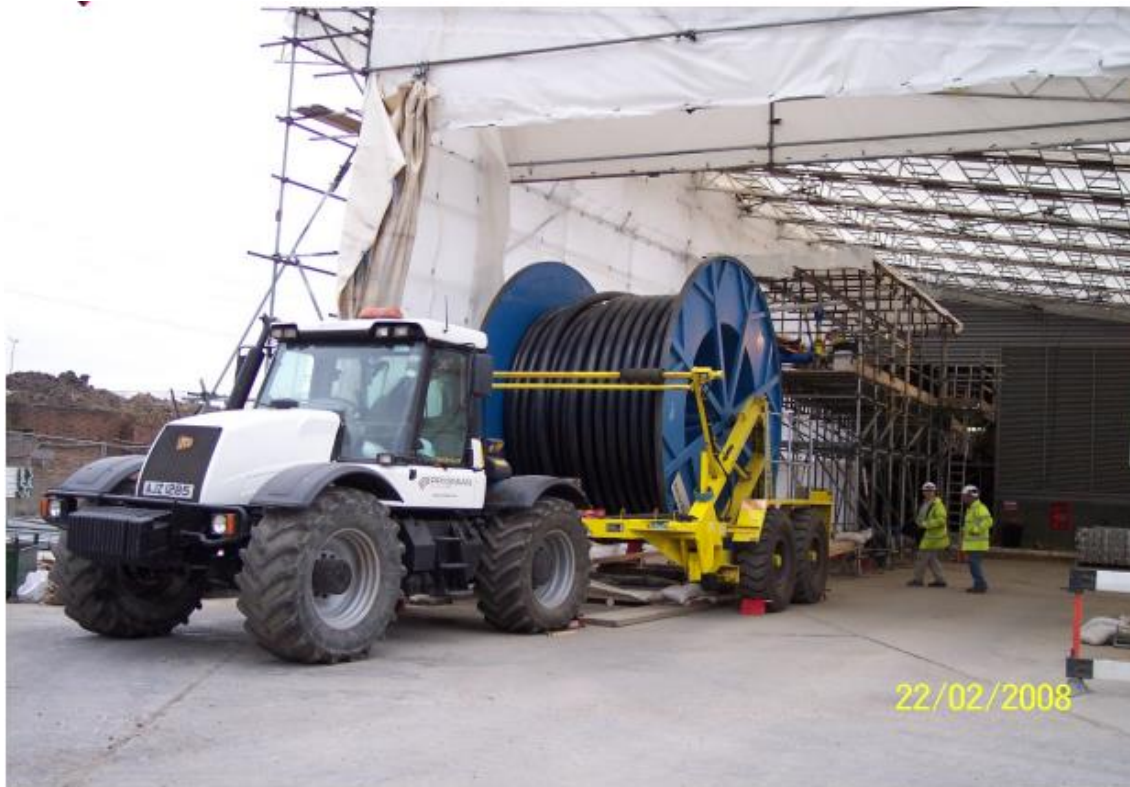
Figure F.8: Cable winching from drum
