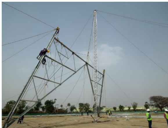
Figure D.15: Erection using derrick pole
