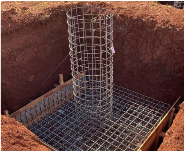
Figure D.12: Pad and chimney foundation
