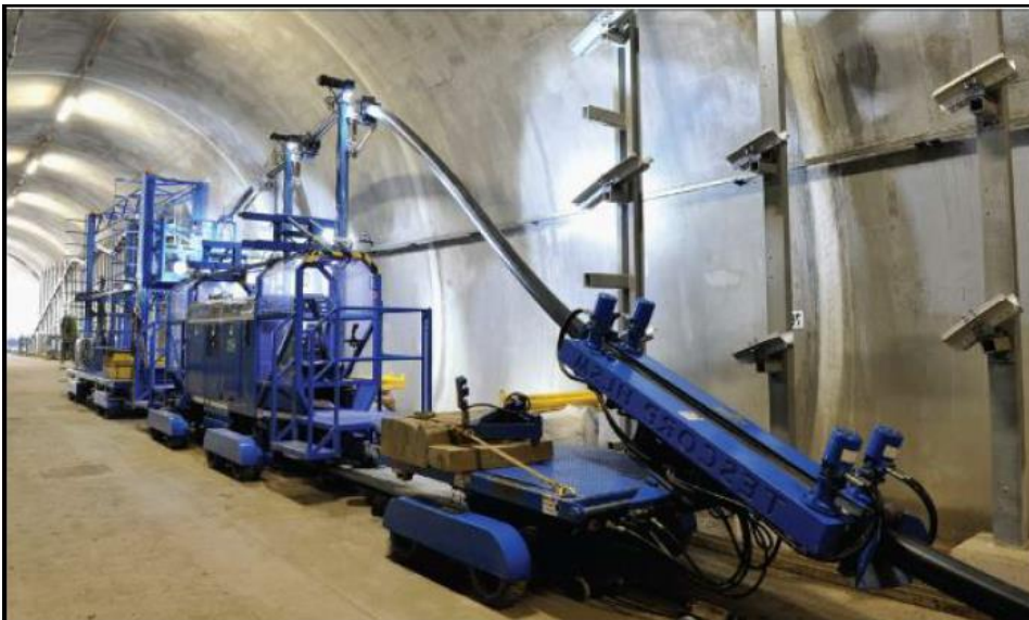
Figure F.10: Automated tunnel cable installation machine
