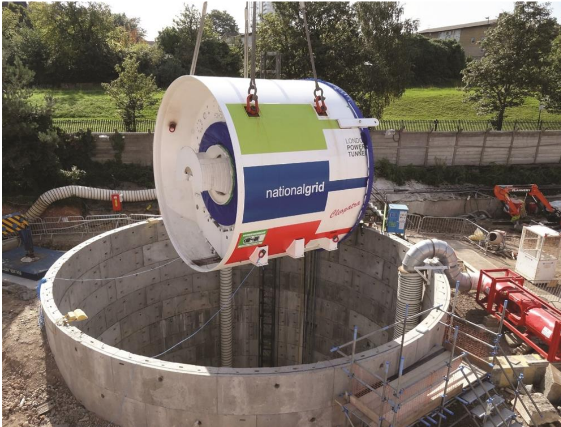
Figure F.2: Tunnel shaft insertion
