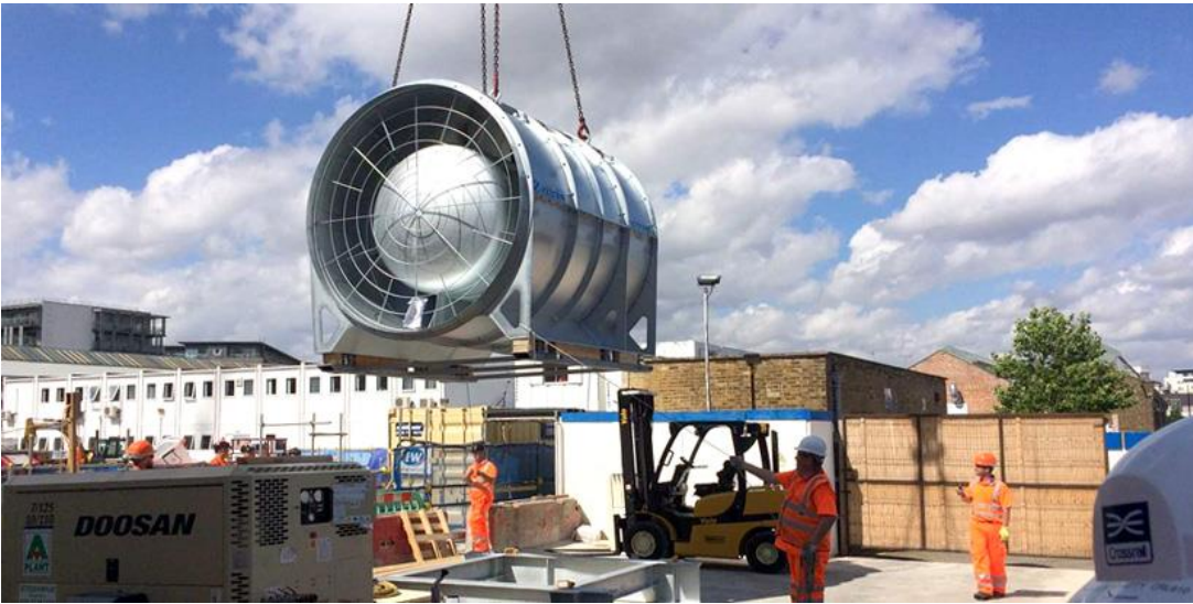
Figure F.5: Tunnel ventilation system installation
