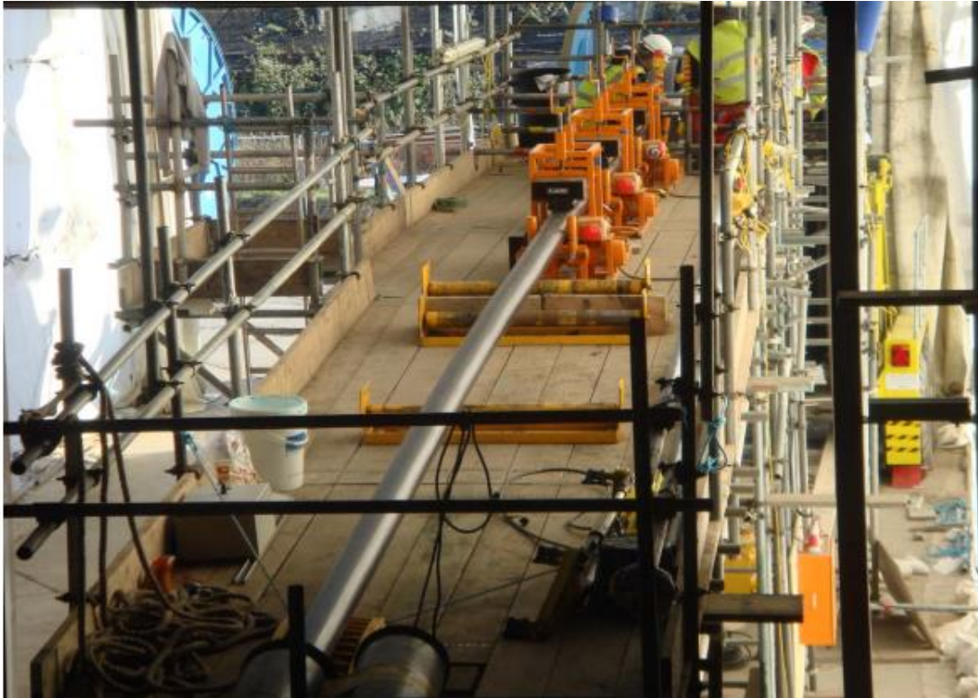
Figure F.9: Cable being lowered into tunnel
