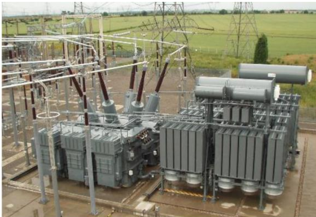
Figure H.4: Example of a quadrature booster at NGET's High Marnham substation
