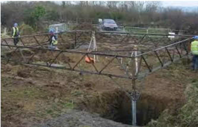
Figure D.11: Foundation setting template
