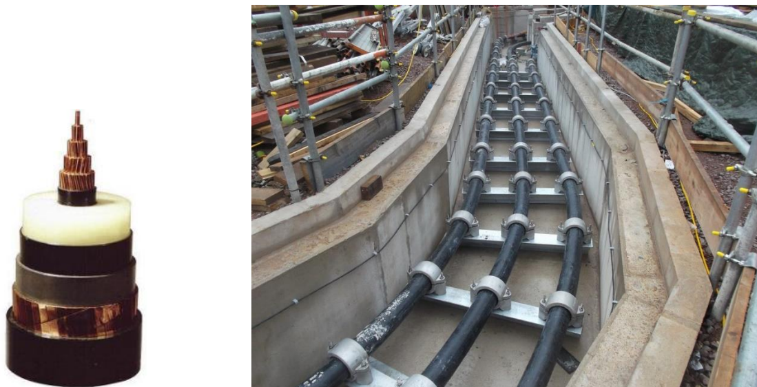
Figure 2.4: a) Typical UGC, b) UGC Installed in Trough
