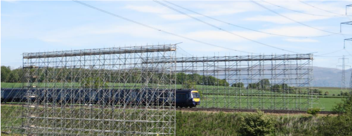
Figure D.10: Scaffold protecting railway line
