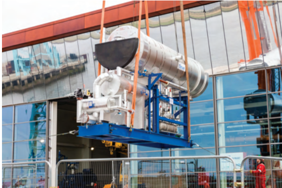
Figure 18 Installation of 2.65 MW WSHP to power the Clydebank district heating network in Glasgow [3.31] Image courtesy of Vital Energi
