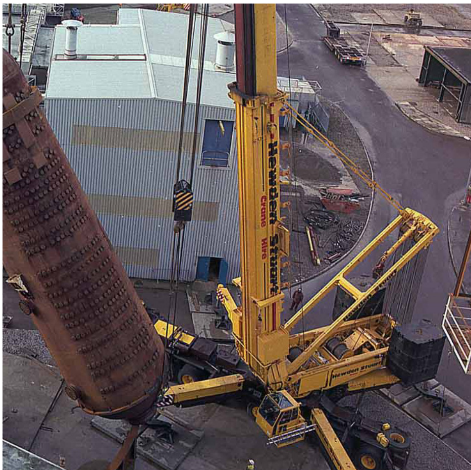
Removal of one of the sealed boiler vessels at Berkeley Power Station
