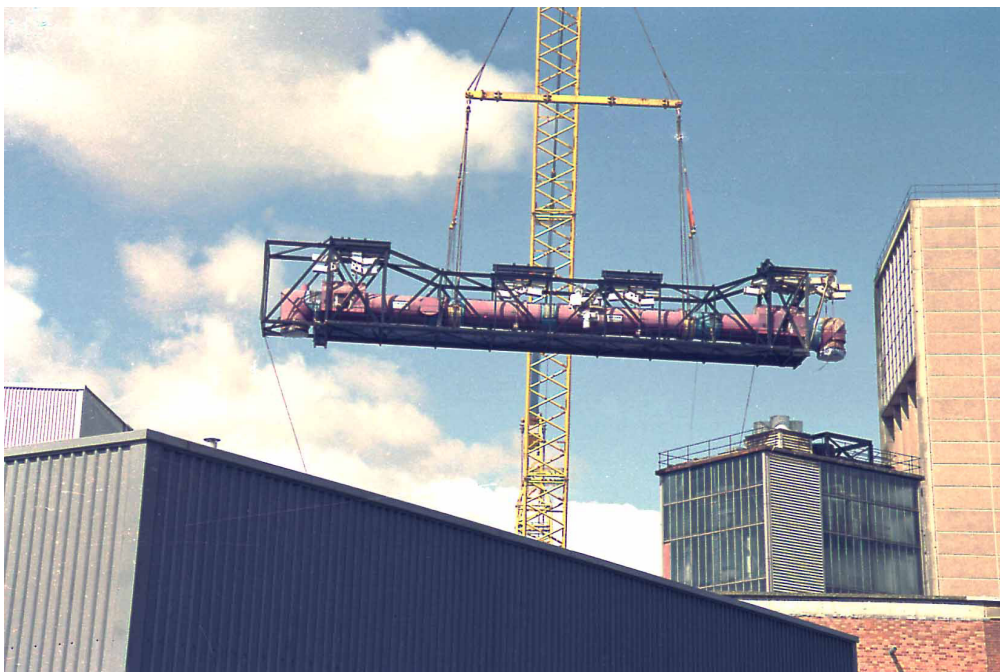
Removal of CO 2 Gas Cooling Ducts at Berkeley
