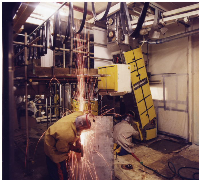
Decommissioning of cubicle 3 gloveboxes in the redundant PFR Plant at Sellafield
