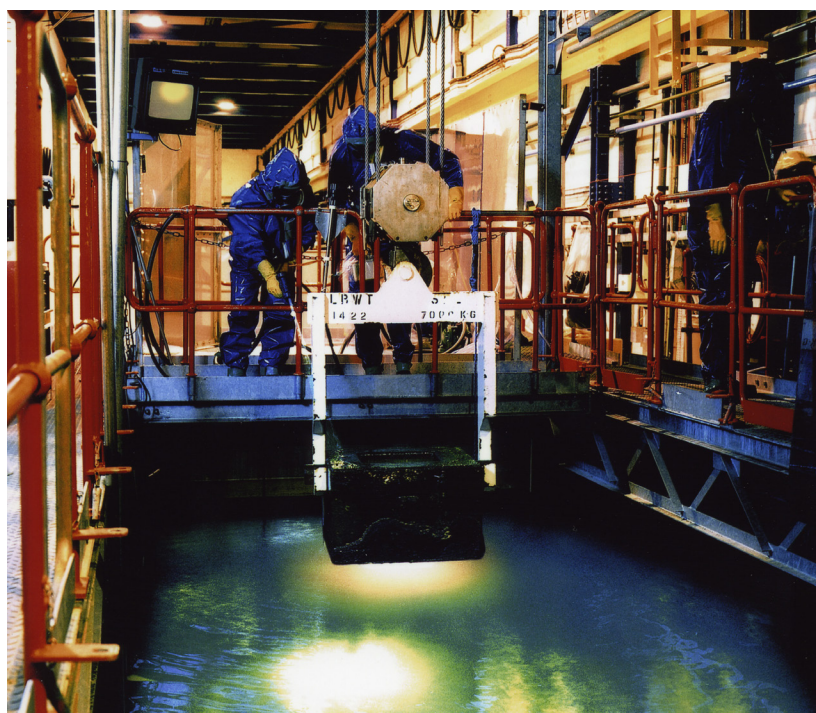
Operators remove a redundant uranium storage flask from the storage pond withdrawal bay at Sellafield
