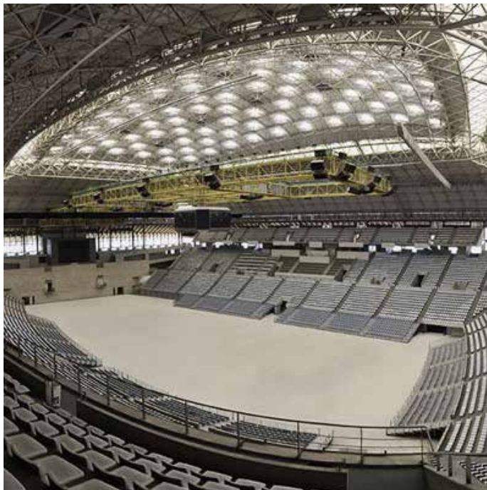
Figure 3 – Interior view of Palau Sant Jordi and structural sensor map
