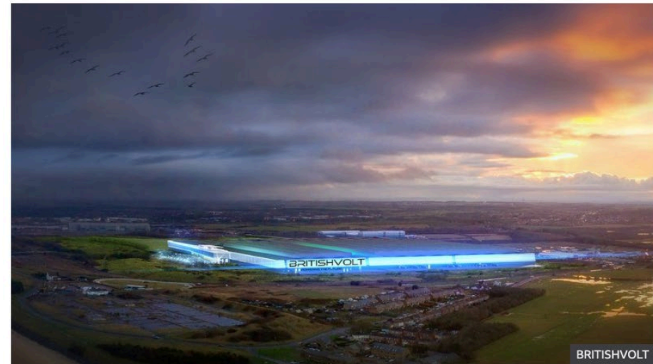
Construction of the "gigafactory" on the site of the former Blyth Power Station is due to start in the summer
