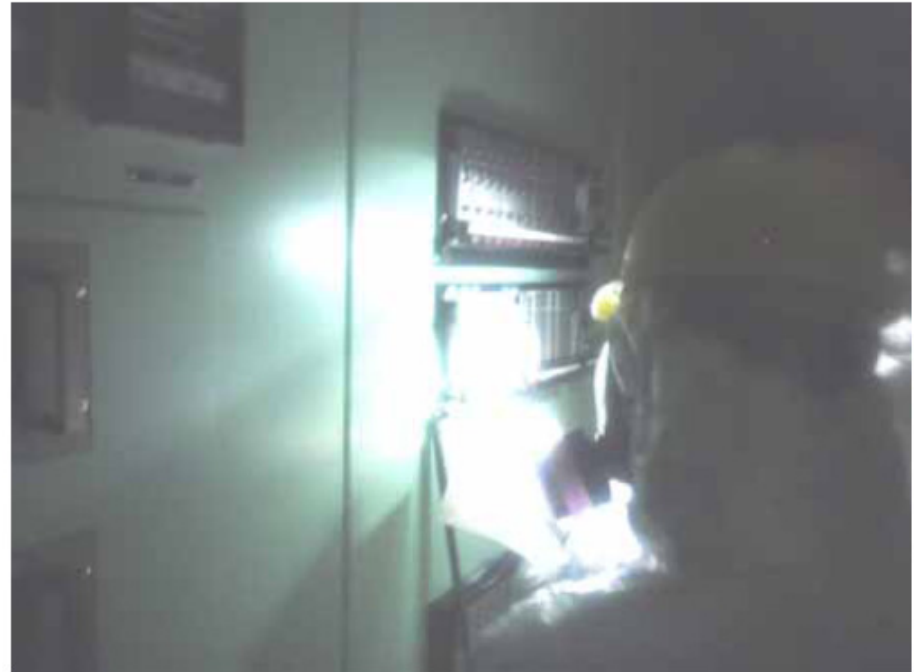
Main Control Room before the lights turned on Checking a meter gauge with a flashlight in darkness•
