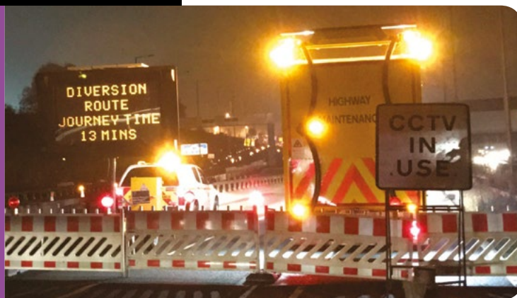
Image courtesy of Rennicks UK Ltd
